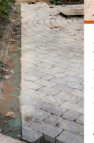
Straight runs are easy. Snap a chalkline, then use a cutoff saw with a diamond blade to make a quick scoring cut along the top of the paver. Make a final pass, cutting through the pavers and slightly into the sand.
