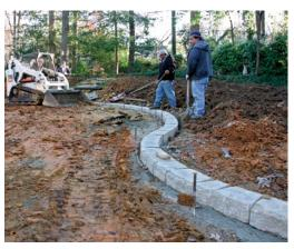
grade pin at this height, and to guard against losing the mark, I wrapped duct tape at the same height. At the patio's far end, I drove another grade pin and stretched a string between the two pins. Measuring down from the string tells whether the soil below is too high, too low, or just right.
