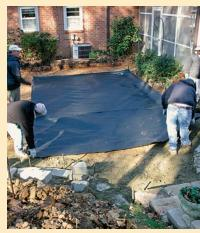
Spread the stone in thin layers. The ABC stone we used for the base includes all gradations of stone from dust to 1½-in.-dia. gravel. This mix can be packed flat and dense without losing its drainage properties. Apply the base in several 2-in. to 3-in. layers, wetting it down to aid compaction. Repeat the layering process until the base is 3 in. from the finished elevation.
