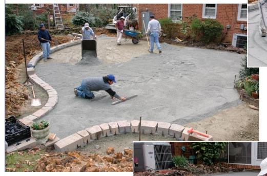
Fine-tune the setting-bed layer. After spreading and compacting the coarse sand over the base, I extend stringlines from the grade pins to identify the finished height of the patio. Then we use a paver and a 4-ft. level (or other straightedge) to fine-tune the setting bed. The final smoothing fluffs the sand a little after compaction so that the pavers bed nicely in the sand.
