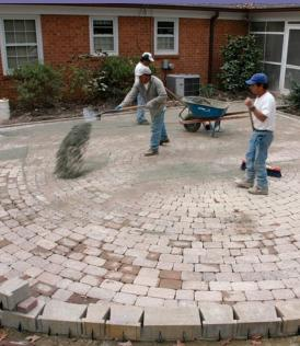
Sweep sand into the cracks. We spread clean, coarse sand over the patio and sweep it into the cracks. Then we vibrate the pavers with a compactor to lock the pavers into place. We repeat the process at least one more time: spread, sweep, and vibrate.
